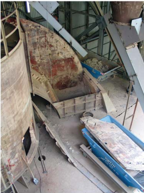
9 Dismantling of the riser duct GL32 Demontage der Gasleitung GL32
